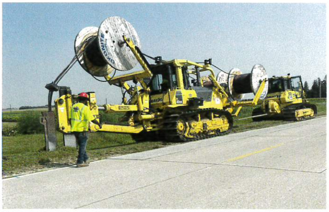
Loosbrock Digging crews bore in the underground wire.
