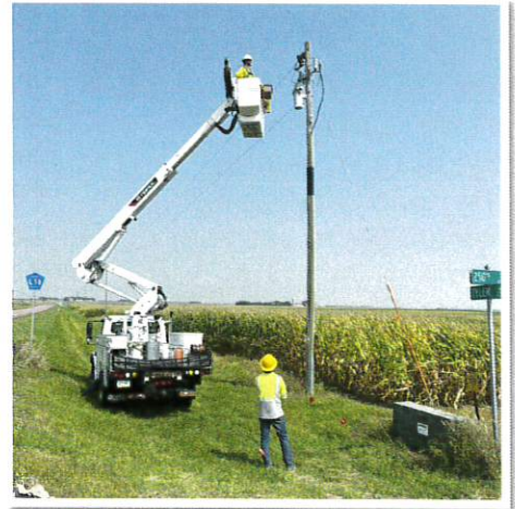
OEC linemen, work with Loosbrock Digging crews to tie in the services.
